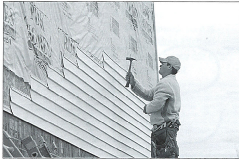
Juan Galvan puts the light beige vinyl siding on the House Chronicles home. Vinyl siding can look cheap or very good, depending on the aesthetics and trim with which it's installed.
